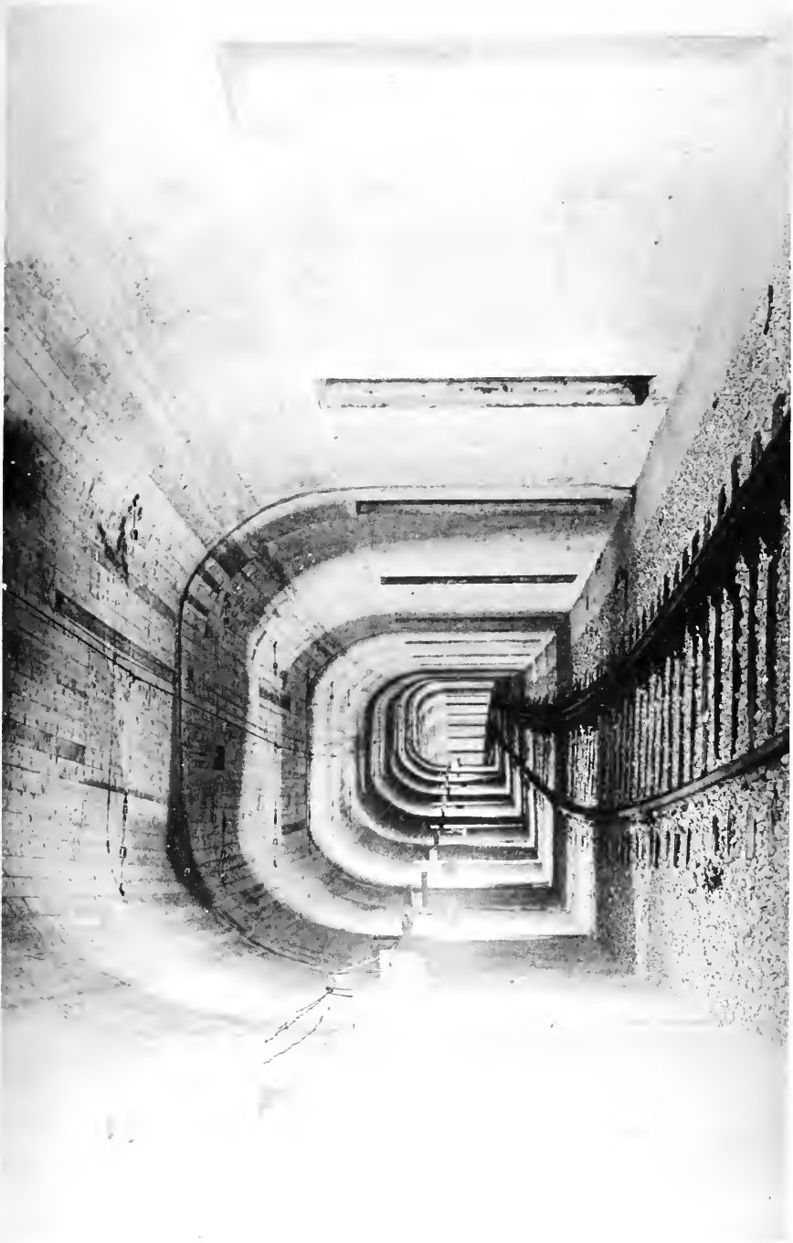
BOYLSTON STREET SUBWAY. SECTION 1, LOOKING EASTERLY, IN SOUTHERLY TUBE, FROM UNDER COMMONWEALTH AVENUE NEAR CHARLESGATE WEST.
